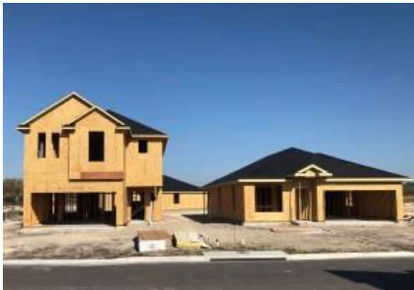
Homes under construction at Legacy.
